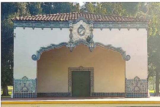
Stage Side Building
